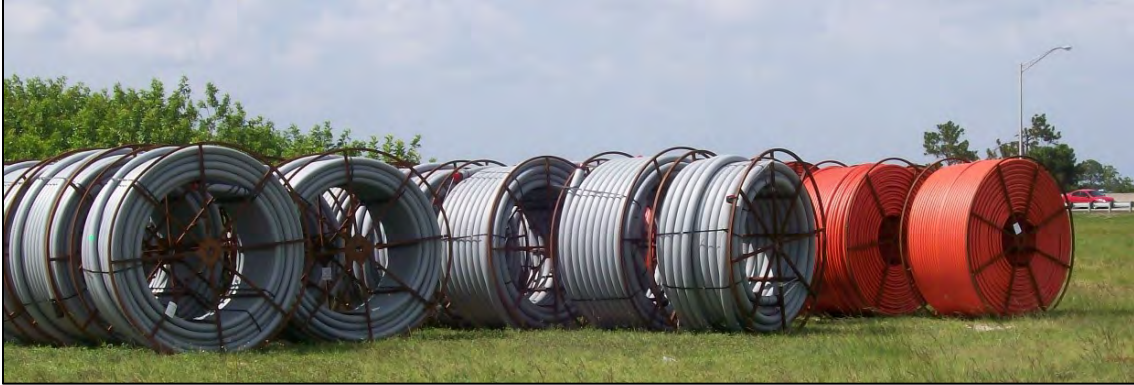
Figure 9. Reels stored vertically on flat, level jobsite.
