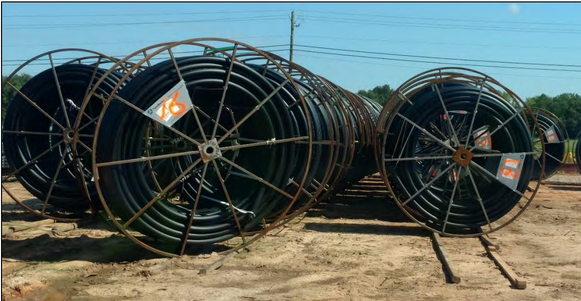
Figure 10. Reels stored vertically on flat, level jobsite.
