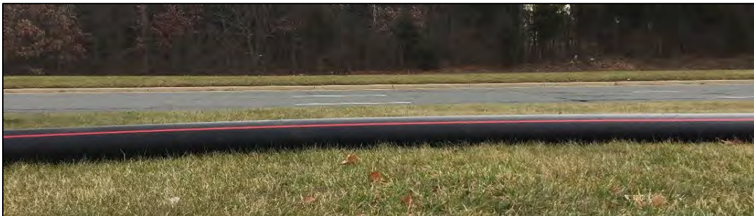
Figure 18. Nominal pipe size 8 PE conduit being laid flat before installation
