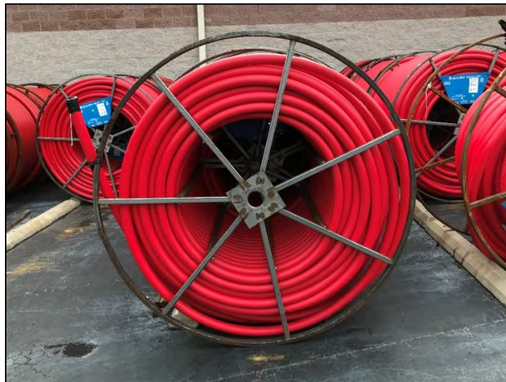
Figure 8. Reels stored vertically on jobsite. Note curbs to prevent rolling.
