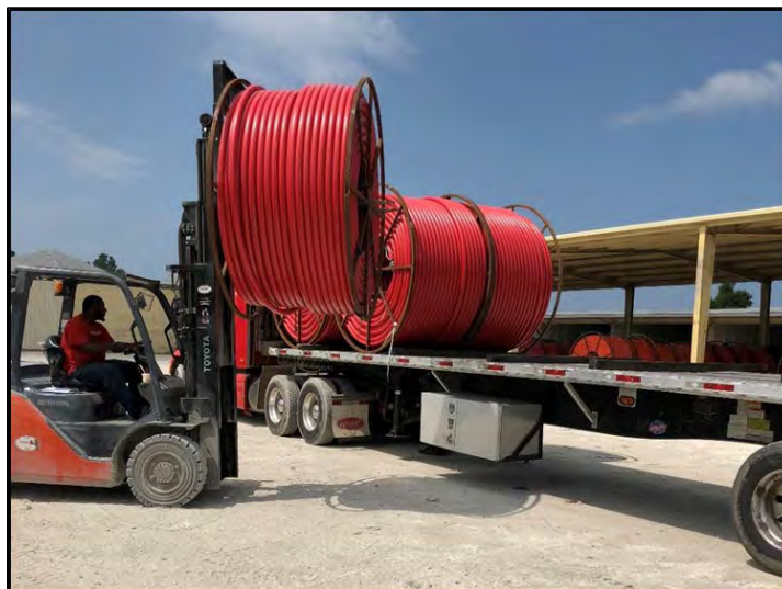
Figure 2. Flatbed truck being unloaded on level ground
